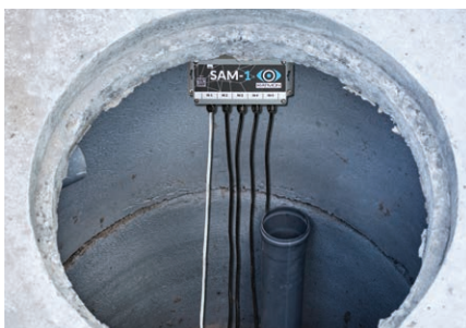
Unit can be mounted inside manhole
